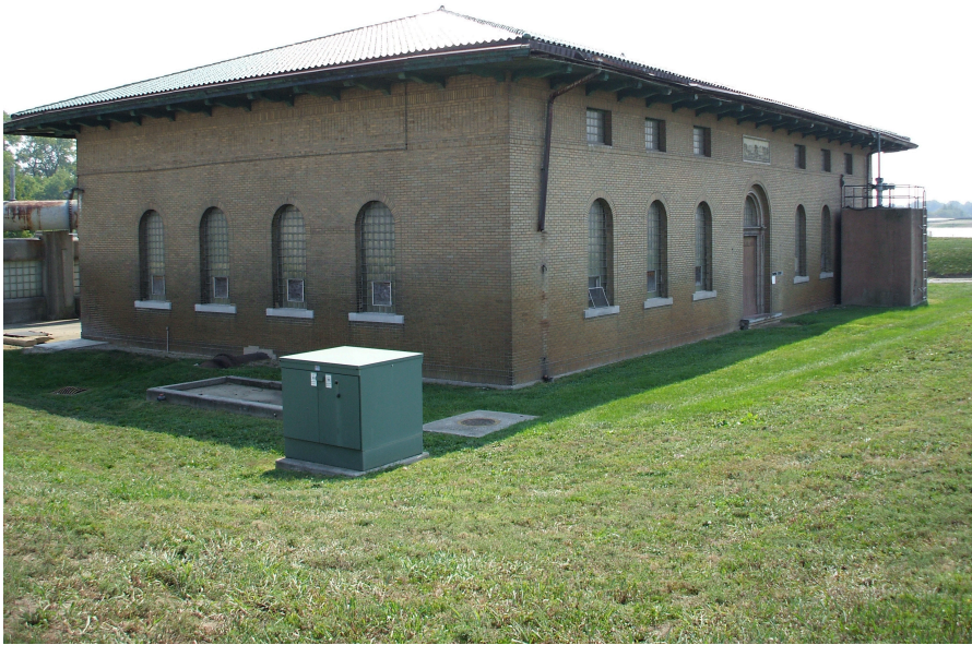
Figure 9. Pump House exterior, Belmont Advanced Wastewater Treatment Plant, 19 September 2007. Photograph by author.
