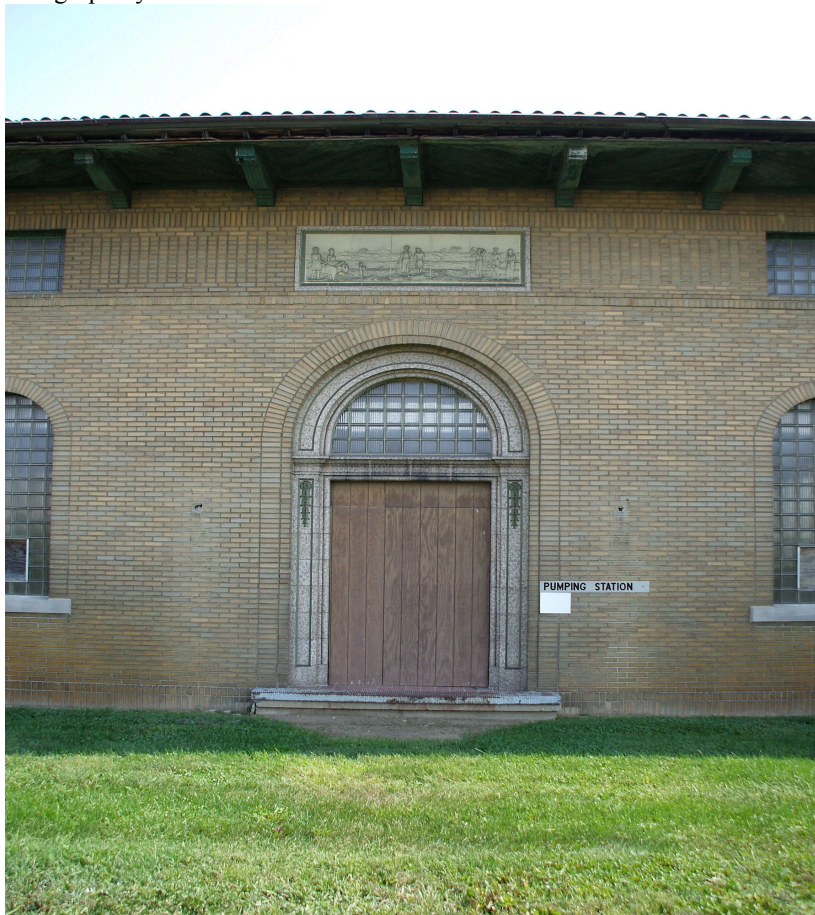
Figure 10. Pump House front view, Belmont Advanced Wastewater Treatment Plant, 19 September 2007. Photograph by author.
